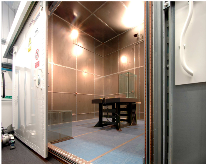
HVTF – High Voltage Chamber
